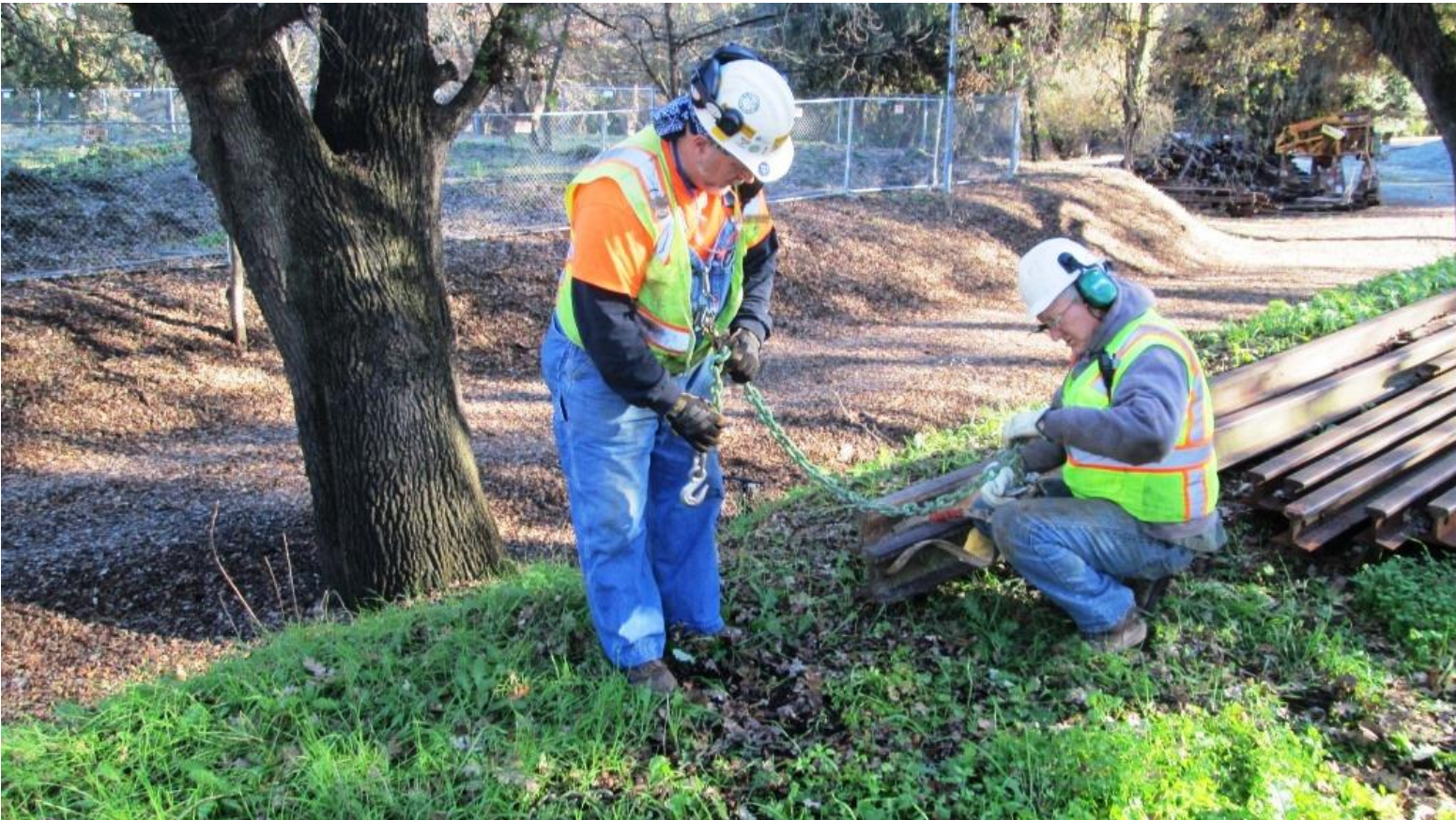
At Front Street, Mike F. and Steve hook a chain to the stick of 110-pound rail to pull it out of the pile
