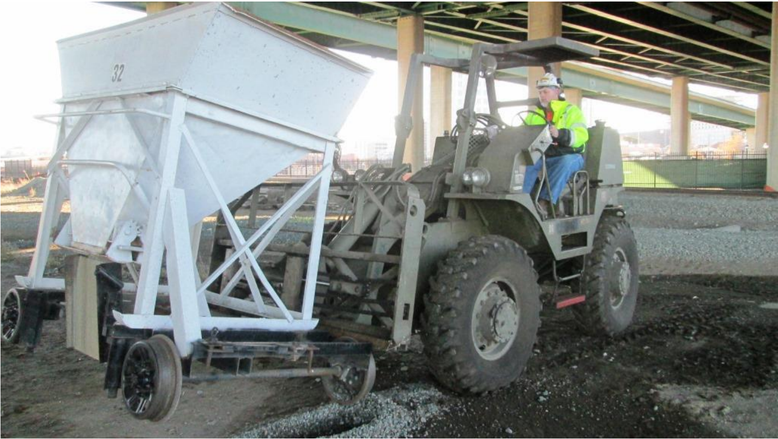
But first, Mike F. uses GM2 to lift the ballast-hopper cars onto the track
