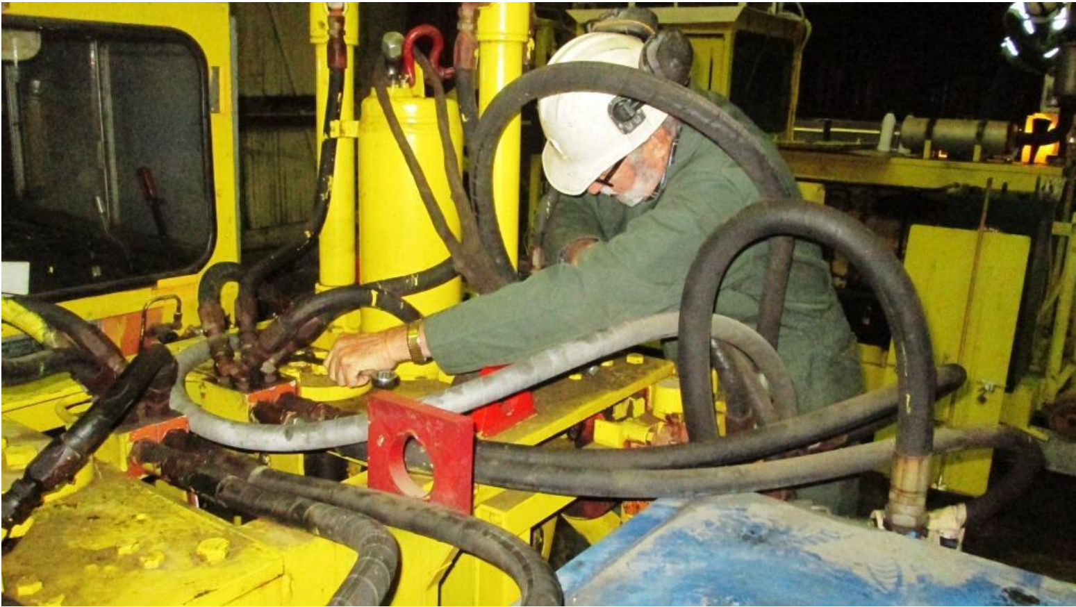
Alan removes the bolts holding the guide-rod for the main shear lift-cylinder in place
