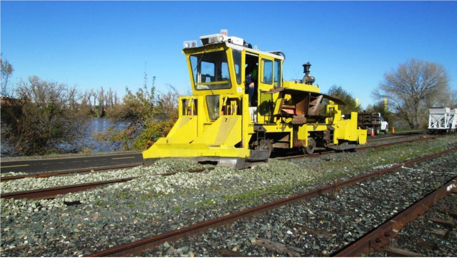
Chris deploys the plows and spreads the rock evenly
