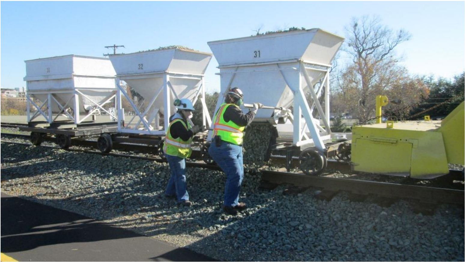
Pam and Heather discharge rock on the west side of the track
