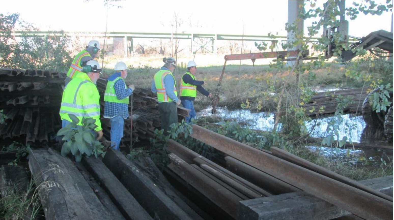
Andrew grabs the rail-tongs from Big Green to connect to one of the 90-pound rails identified by Frank, Steve, Mike M., and Alan
