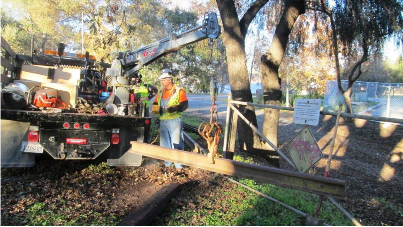
Mike F. maneuvers the crane to load the cut piece into the truck
