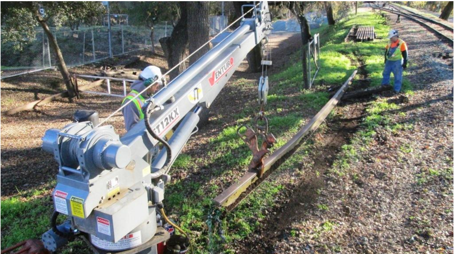
At the controls of the crane, Steve lifts the rail as Mike F. shoves a piece of old tie beneath it
