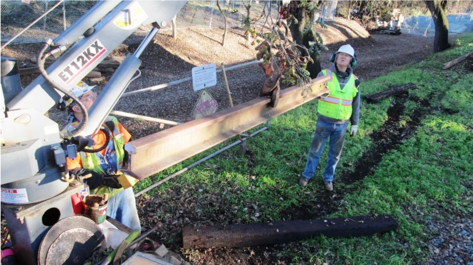
Steve guides the cut rail around low-hanging branches as he and Mike F. load the rail into the truck
