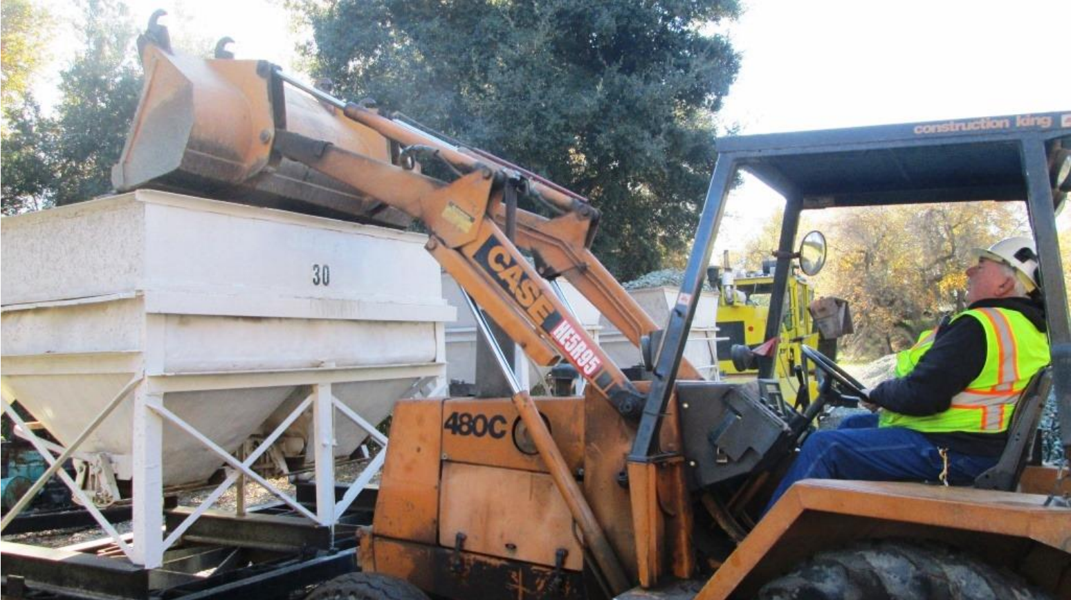
Harry fills the center-dump hopper with rock
