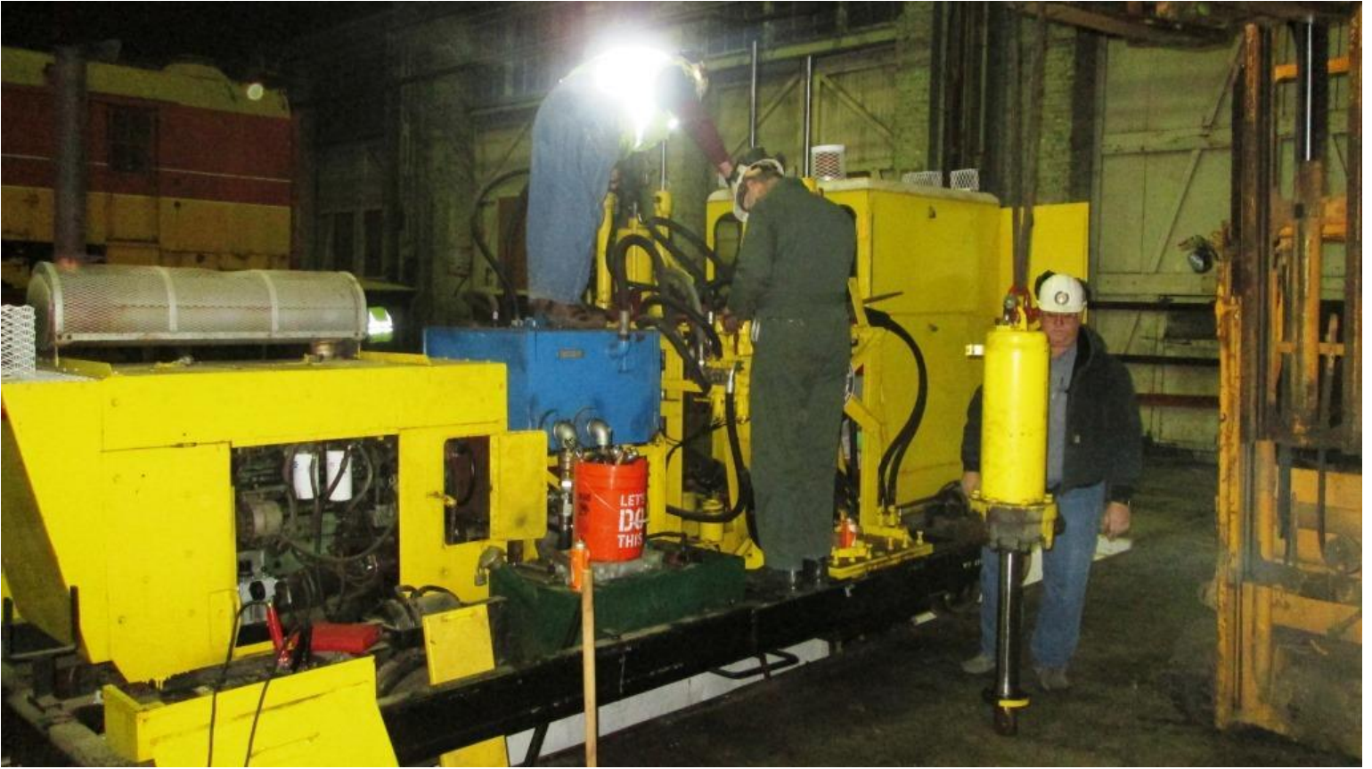
The lift-cylinder is out. It only weighs about 500-pounds...
