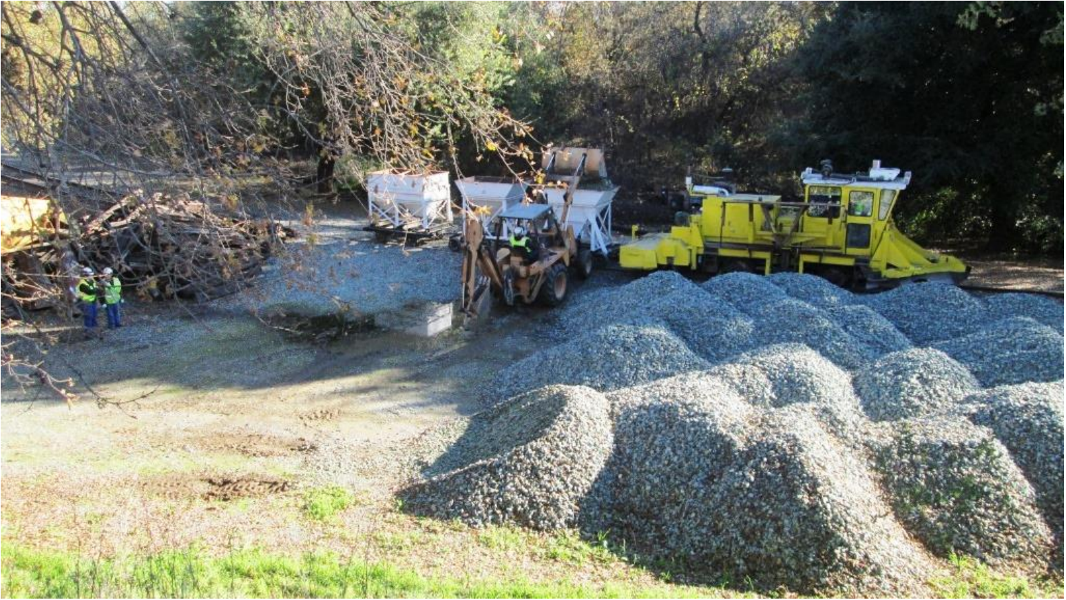
Meanwhile, down at Setzer, Harry on the back-hoe loads the side-dump hopper with ballast-rock
