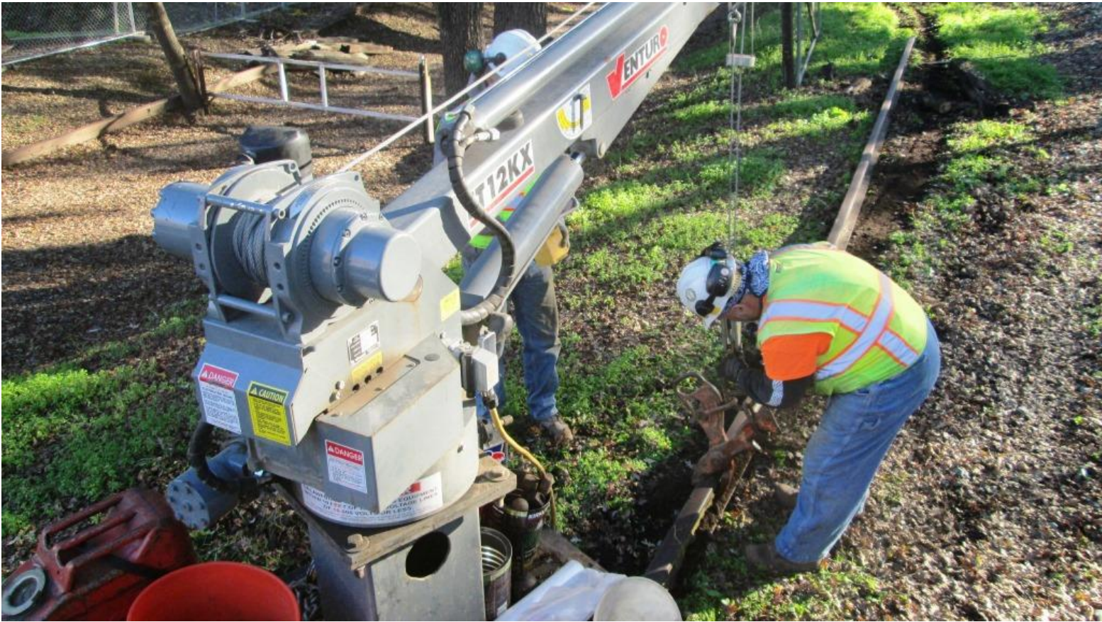
Mike F. attaches rail-tongs to the truck's crane to lift the rail sufficiently to place cribbing beneath it
