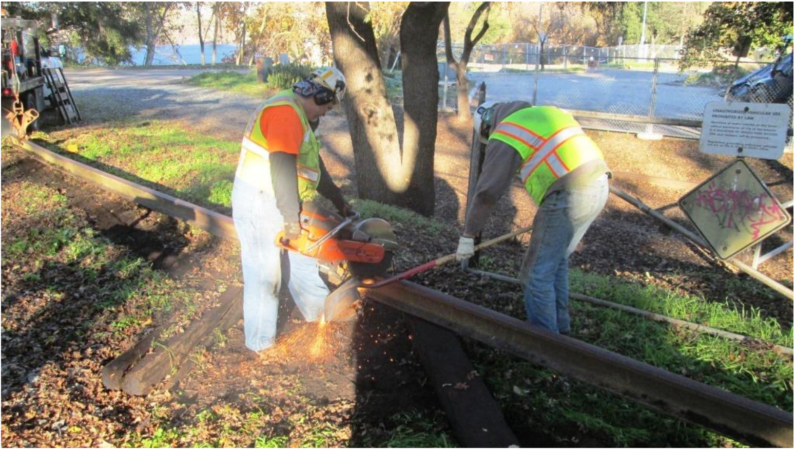
Sparks fly as Mike F. begins cutting the rail. Steve uses a shovel as a spark-shield
