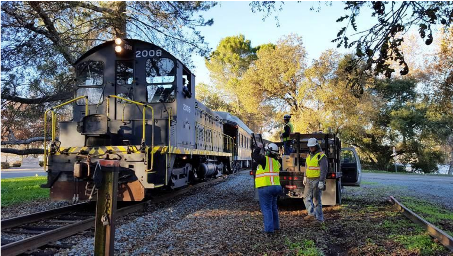
Heather waves to the Polar Express as it passes our work site on its way south to the North Pole
