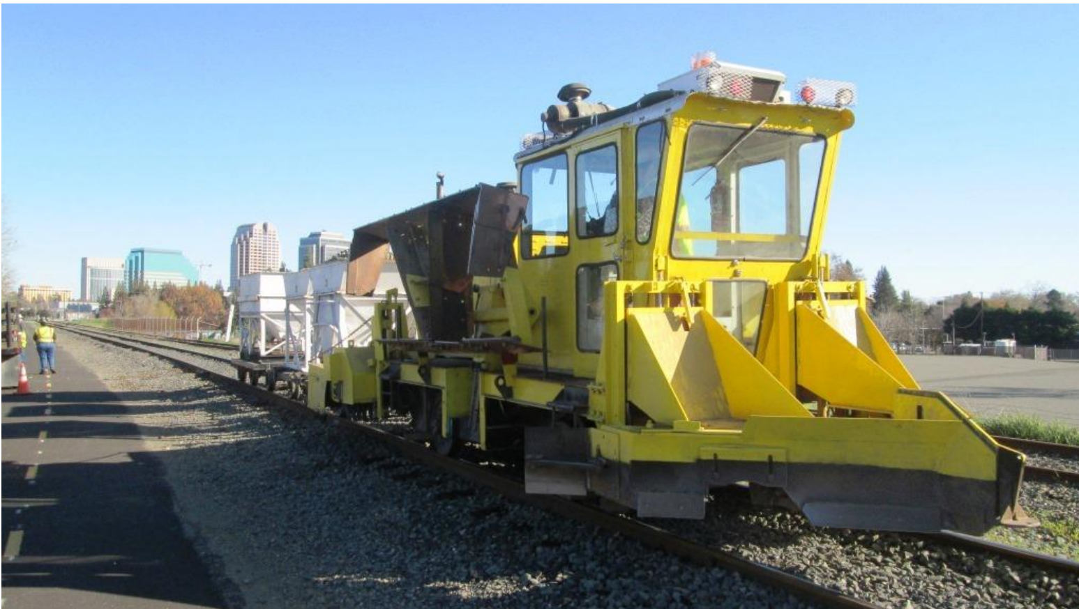
Near Mile Post 1, the ballast regulator is ready to start spreading ballast
