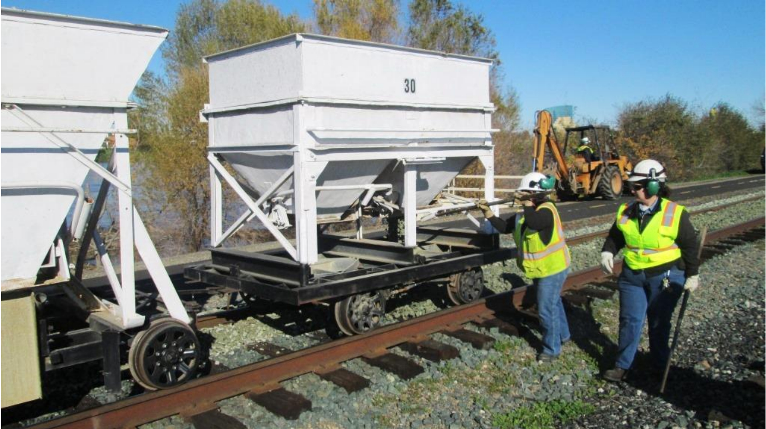
Now Pam drops ballast rock down the center of the track
