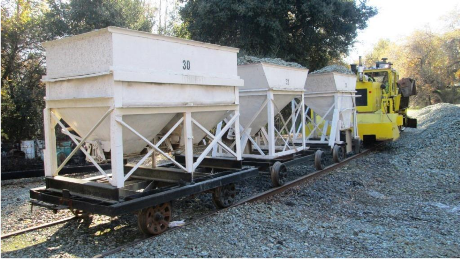
Chris and Anthony in the ballast-regulator pull the filled hoppers up the hill
